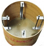
Concrete Form with Anchor Bolts and Rebar
